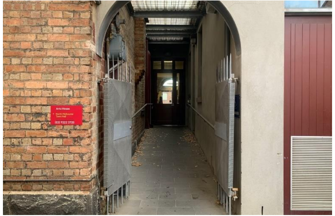
Image: view of the ramp with grab rail leading from George Johnson Lane to the automated door which opens into the Arts House foyer.
