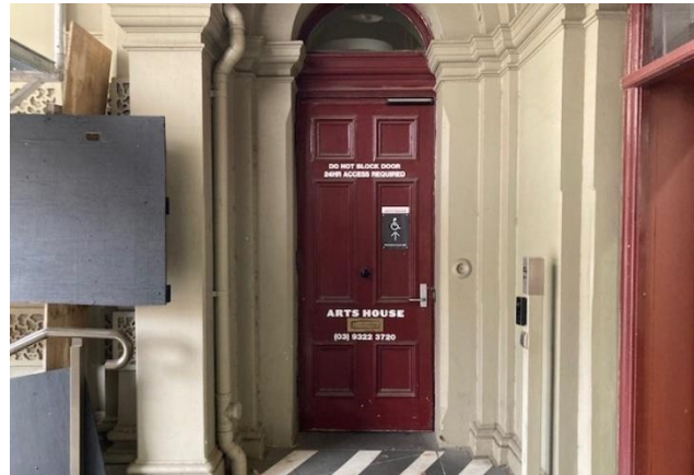
Image: View of door at Post office entrance. Button to open automated door is on the right.
