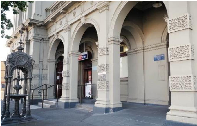
Image: Errol Street entrance next to the Post office with wheelchair accessible ramp or two steps with grab rails.
