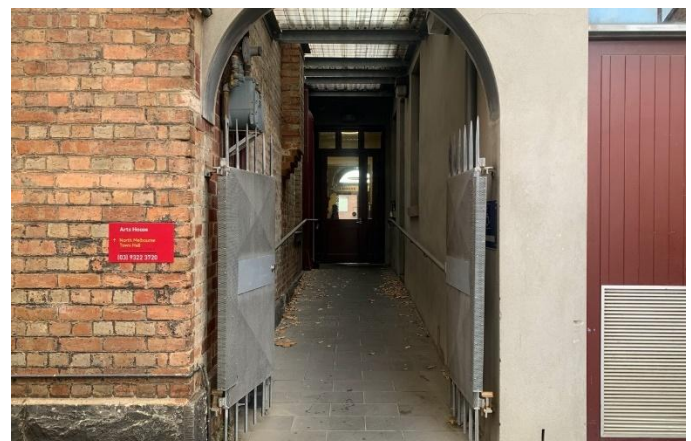
Image: view of the ramp with grab rail leading from George Johnson Lane to the automated door which opens into the Arts House foyer.
