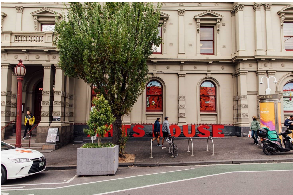
Image: North Melbourne Town Hall entrance on Queensberry Street. The entrance is to the left of the giant red letters that say ARTS HOUSE and features a staircase of eight steps with grab rails in parts.
