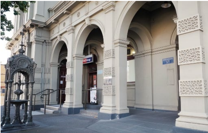
Image: Errol Street entrance next to the Post office with wheelchair accessible ramp or two steps with grab rails.
