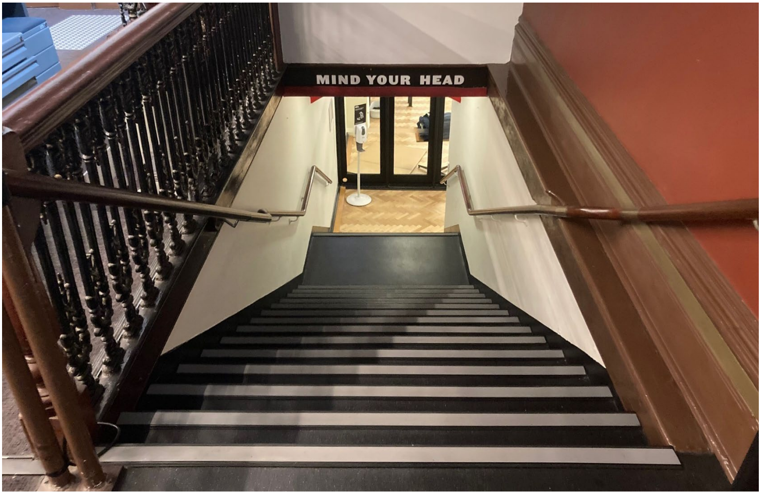
Image: There are 20 stairs with grab rails either side.
