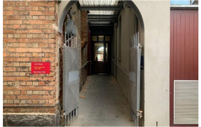
Image: view of the ramp leading from George Johnson Lane to the automated door which opens into the Arts House foyer.
