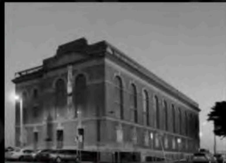
The Substation 1 Market St Newport
